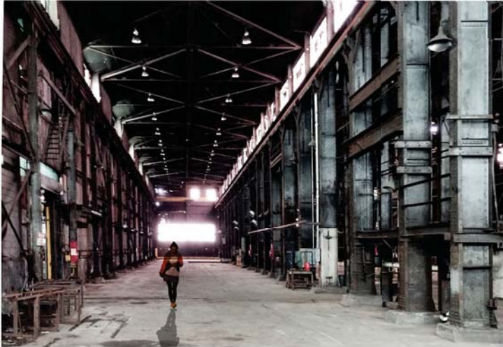
BAY 4 TODAY, REMNANTS OF PHOENIX ROLLWORKS
