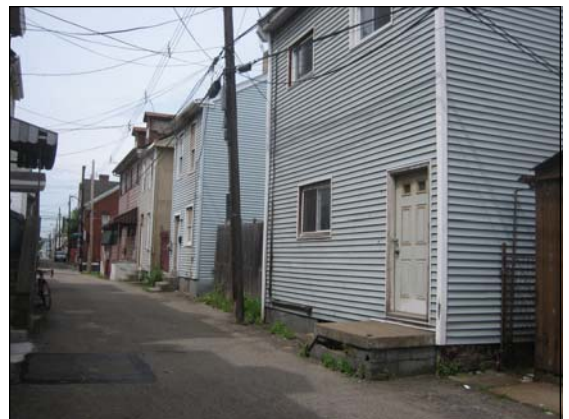
Houses on Dresden Way slated for demolition
